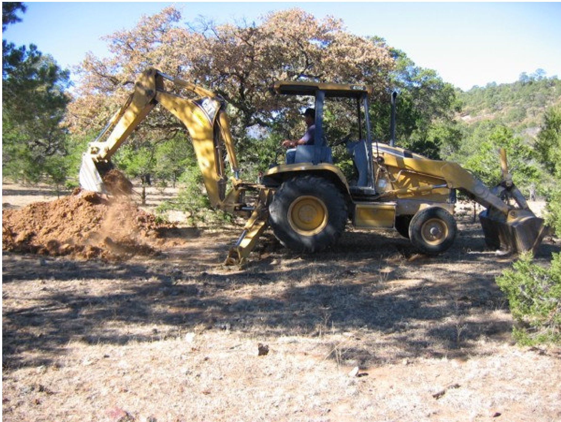
Trenching at Sandra Project
