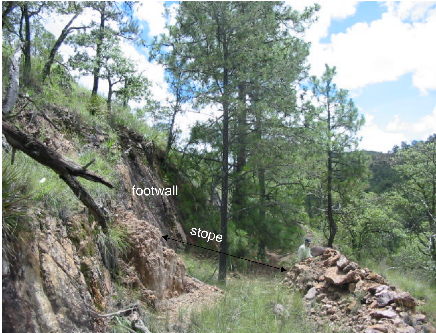
Looking SE: several pine trees have grown on the collapsed open stope. The width of the mine workings is around 4.0 meters.
